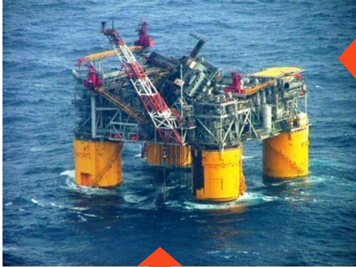
Mars drilling rig collapse (GoM in hurricane Katrina, 2005)
