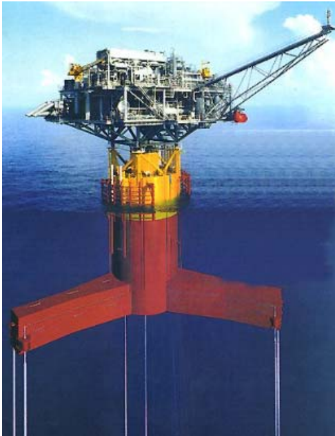
SeaStar TLP installed in 1998
