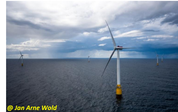
HYWIND Scotland 30 MW (5 FOWT of 6 MW– October 2017)
