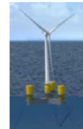
Groix – Belle Ile Developer: Eolfi/CGN 4 x GE 6MW turbines Floater Naval Energies (demonstrator)
